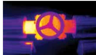
Thermal camera view of the uninsulated valve
